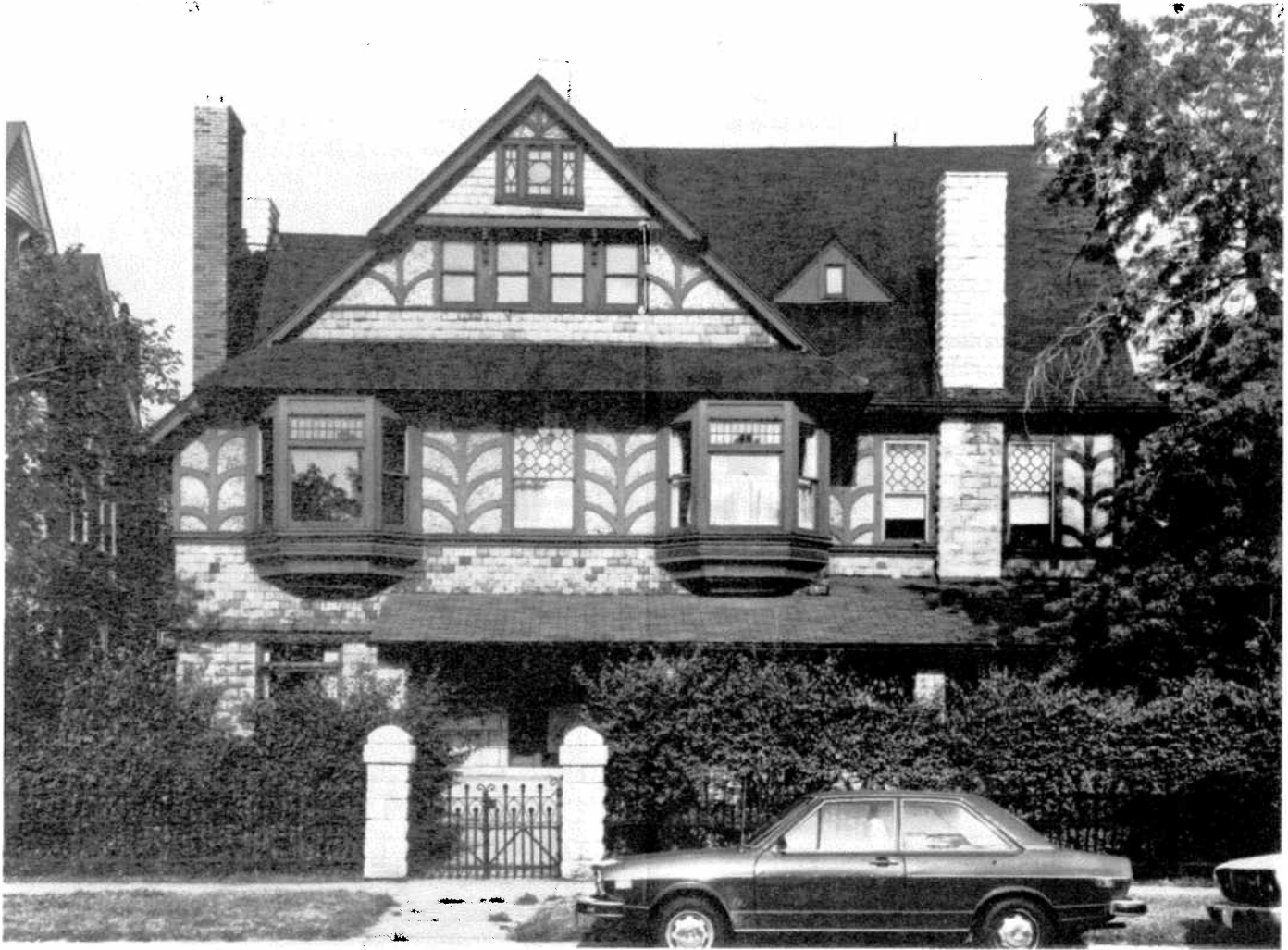
This house at 4800 Kimbark Avenue was built around 1888 and is an excellent example of the Queen Anne style. The facade is arranged more formally than those of most Queen Anne houses. A variety of materials of different colors and textures enlivens the facade, and projections, chimneys, and intersecting roofs create a picturesque composition. (Barbara Crane, photographer)
